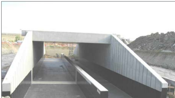
Completed Structure in July 2010
