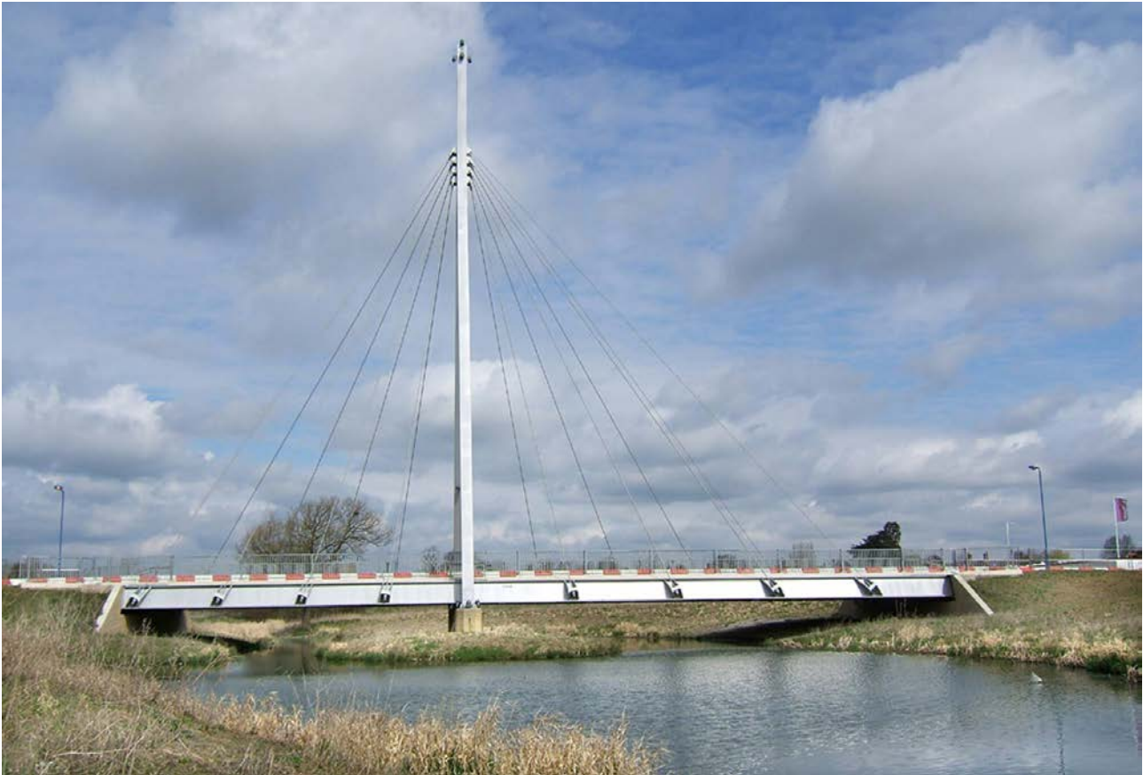
Broughton Cable Stay Bridge
